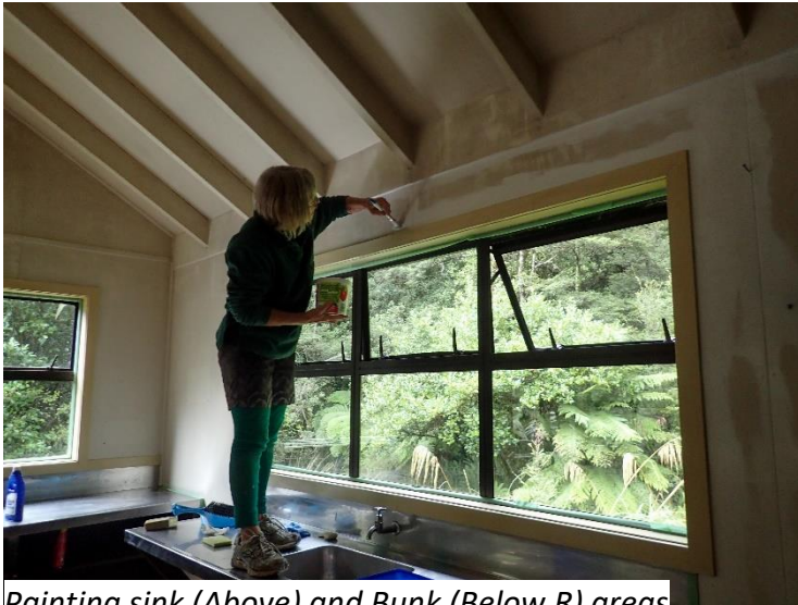
Painting sink (Above) and Bunk (Below R) areas
