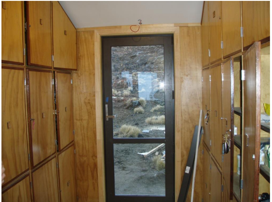
New fire exit door in locker room at the lodge
