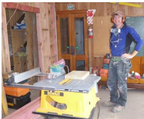
Rob at work on Lodge Lockers
