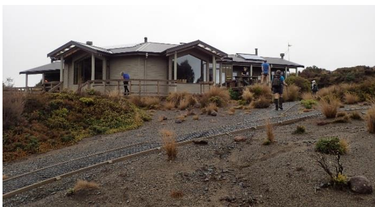
The super flash Waihohonu Hut
