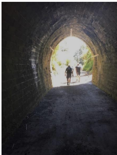
The Long Tunnel (565m)
