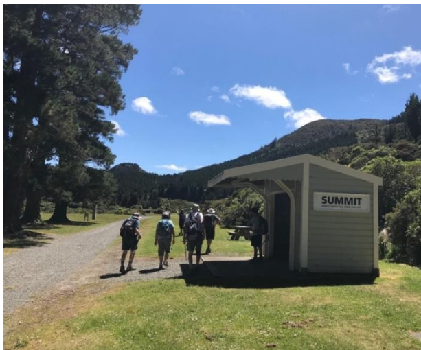
The Summit Station at 1141feet above sea Level
