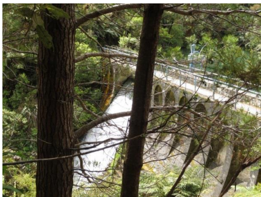
View of the dam
