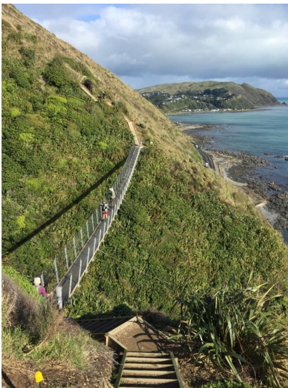
One of the Escarpment Superior Swing Bridges
