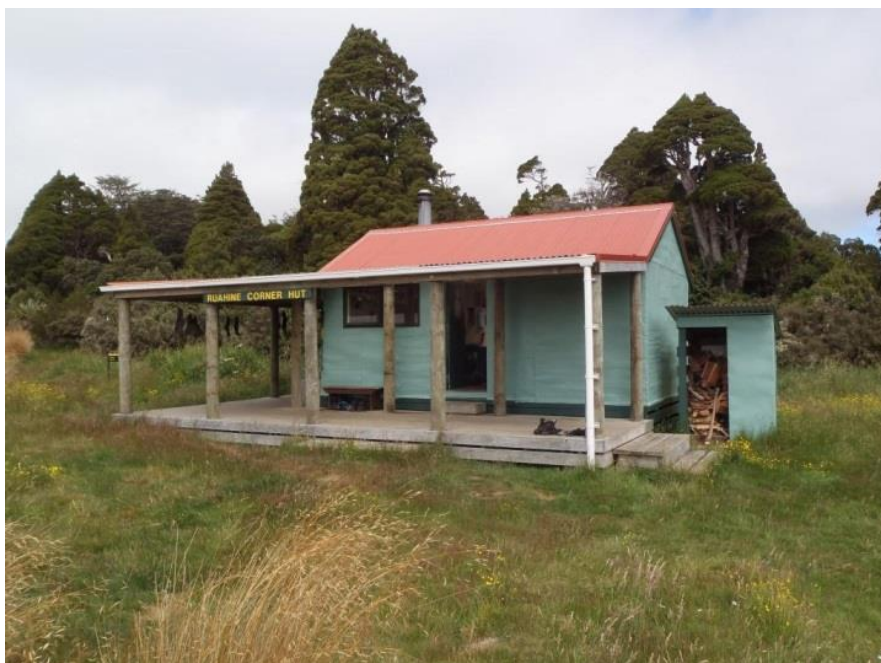
Ruahine Corner Hut
