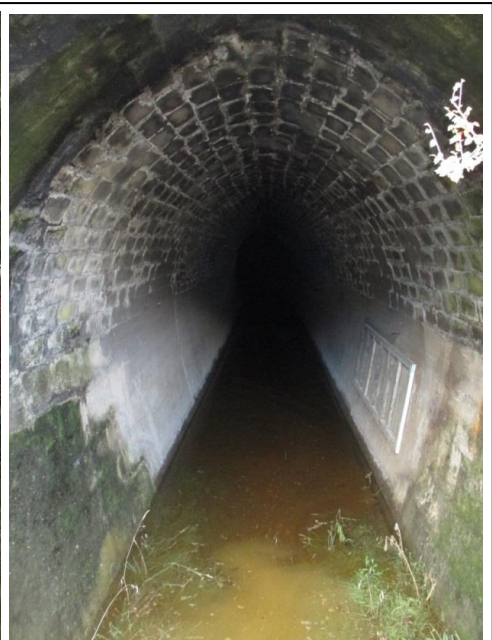
Old railway tunnels, need a canoe!!
