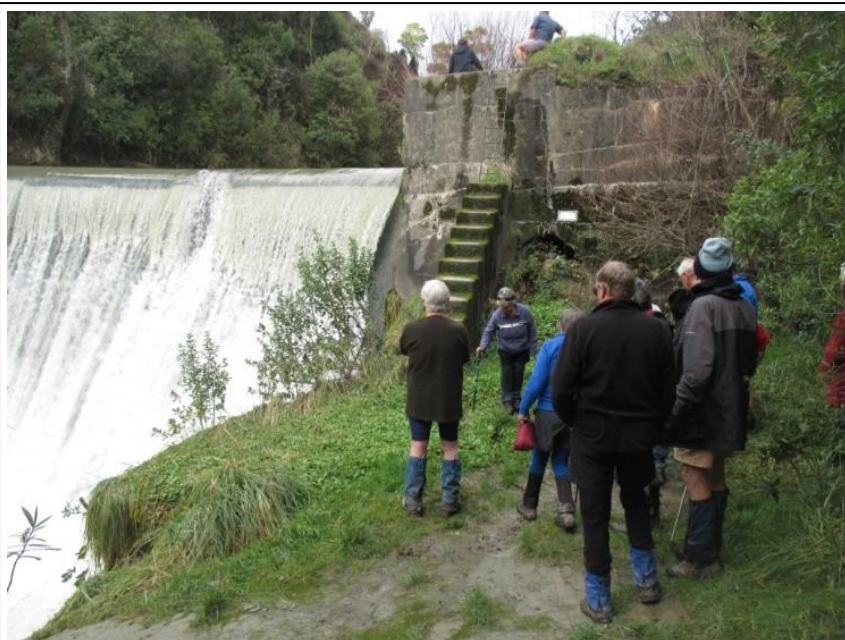
Mangaweka 1911 power station dam and reservoir
