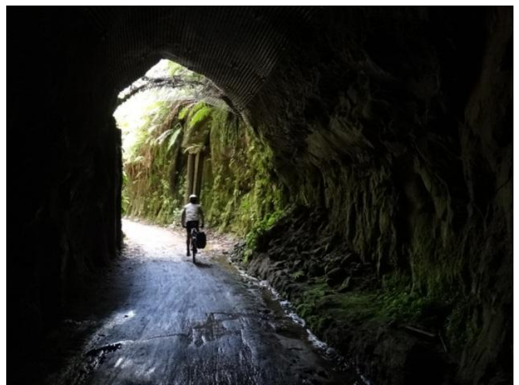
Ken Mercer pedals out of the gloom of the Ongarue Spiral tunnel. DOC has made a big investment here by diverting the stream which had run through it, and by strengthening the roof. Chris Mercer
