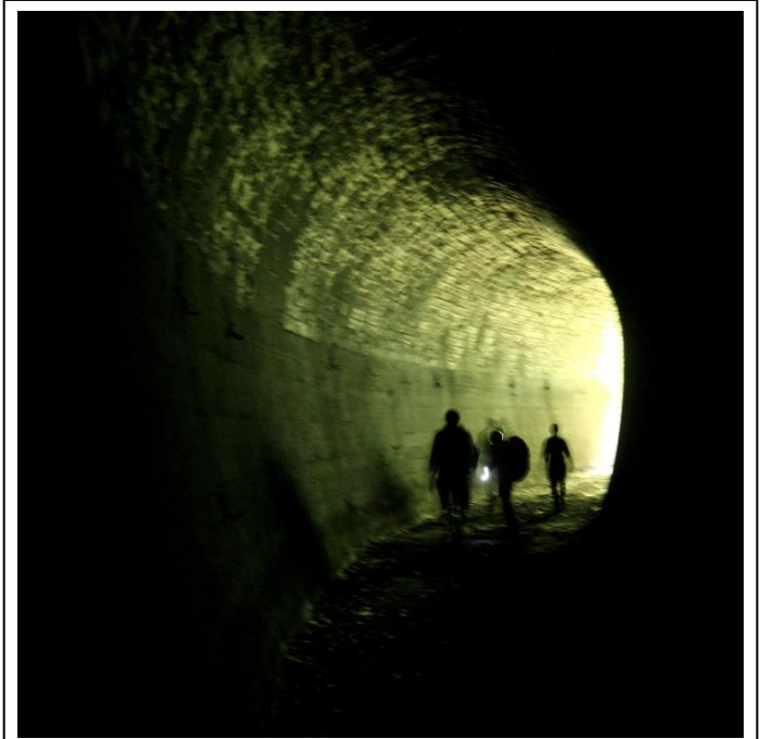
Old Mangaweka Rail Tunnel
