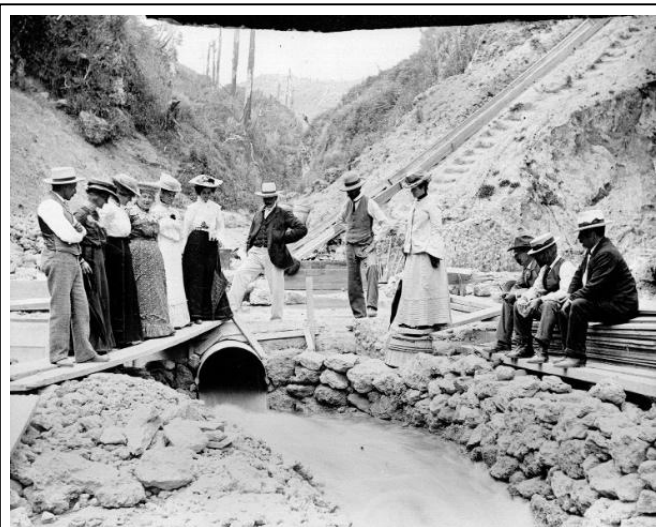
Okehu / Waitahinga dam built in 1904 for water supply to Wanganui. Royce Mills
