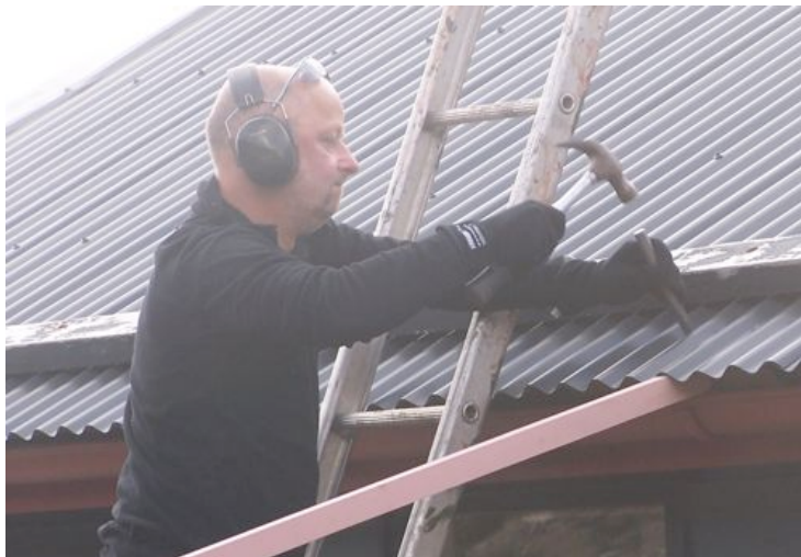
Roger Athersuch punching holes in the Lodge roof: photo Ken Mercer.
