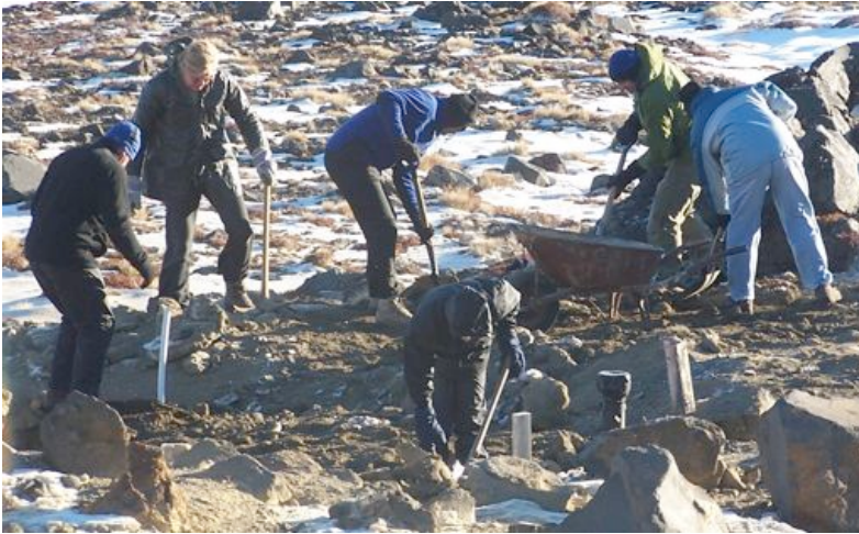
Covering up the Septic Tank
