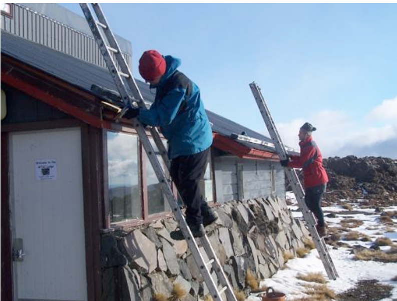
Working on the Lodge roof: photo Ken Mercer
