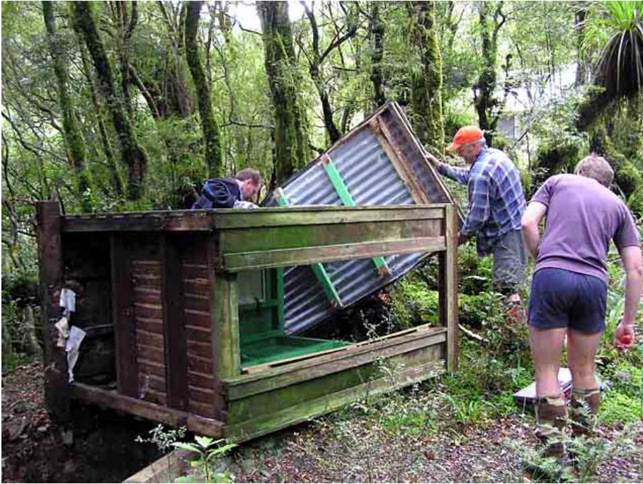
Above: Demolishing the toilet at Mangahao Flats (Photo: Jean Garman).
